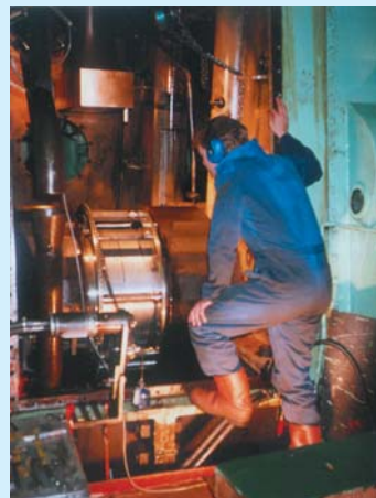
Picture shows a Large Crank Pin being Orbital Machined in Situ.
